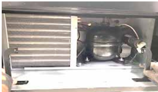
Figure 26 – Refrigeration deck removal
